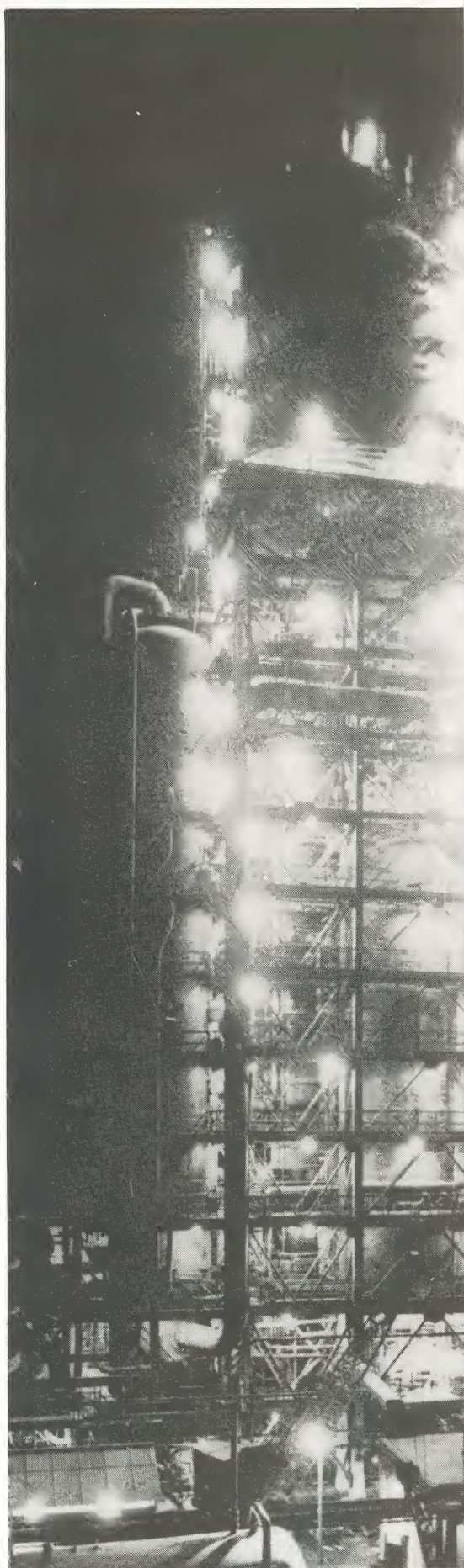
Lago's catalytic cracking unit.
